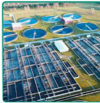
ETP / STP / WTP SYSTEMS
