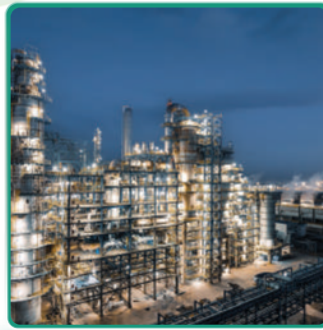
CHEMICAL SUPPLY SYSTEMS
